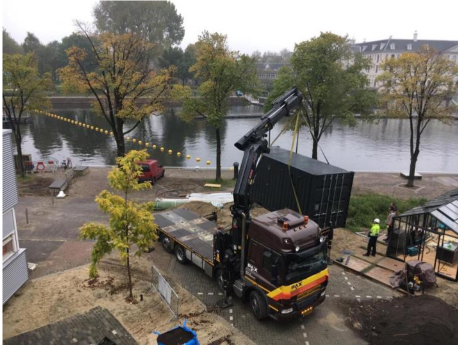
Figure 13: 20ft high cube shipping container – housing the P recovery demo - being installed at the Marineterrein in Amsterdam (Kattenburgerstraat 5) in early October 2019.
