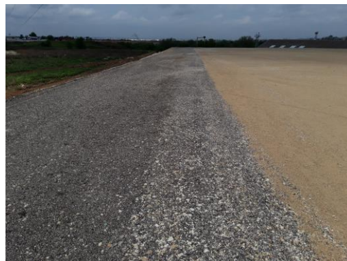
Figure 14: Wearing course manufactured with recycled asphalt aggregates (Source: CINDERELA project)
