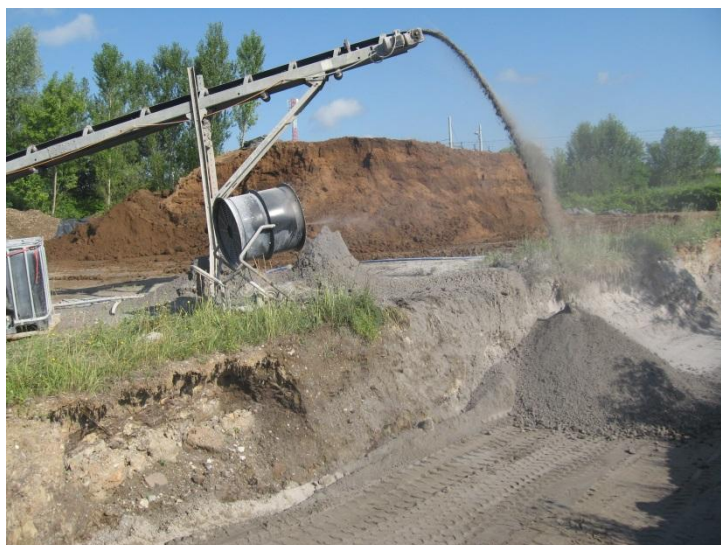
Figure 33: Example of in-situ mixing of binder with waste for production of geotechnical composite
