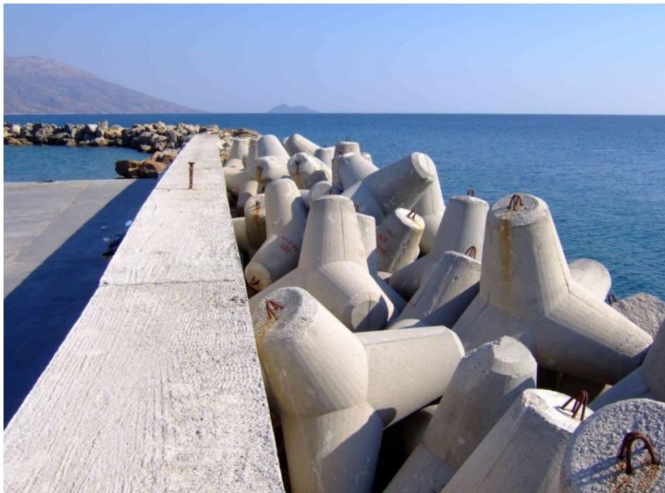
Figure 9: Tetrapods, specialized SRM-based construction products for protection against waves
